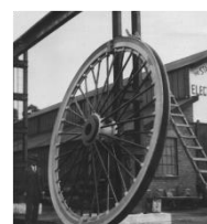
"Doubling-Down" Sheave Arrangement Conveyance Mounted
