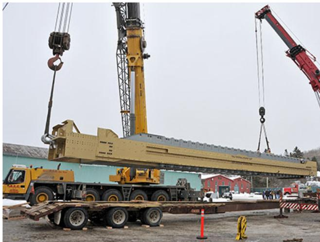
Made of welded steel, each 68-foot high skip is capable of hoisting potash at 4,000 feet-per-minute in the 3,600-foot Vanscoy shaft.
